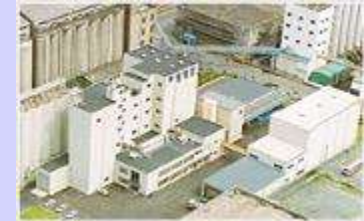
Head Office Plant of Tofuku Flour Mills (Chuo-ku, Fukuoka City)
